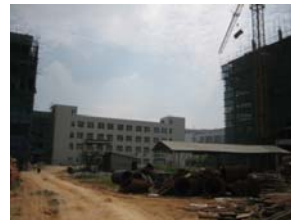
Construction of new manufacturing facility that will double capacity
